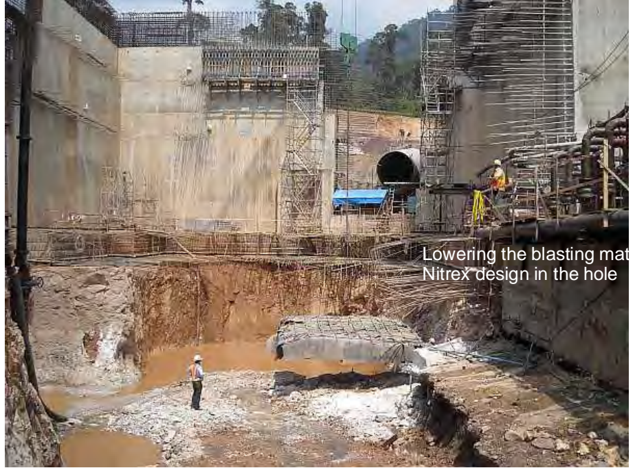
blasting mat Nitrex design in the hole prior to blast
