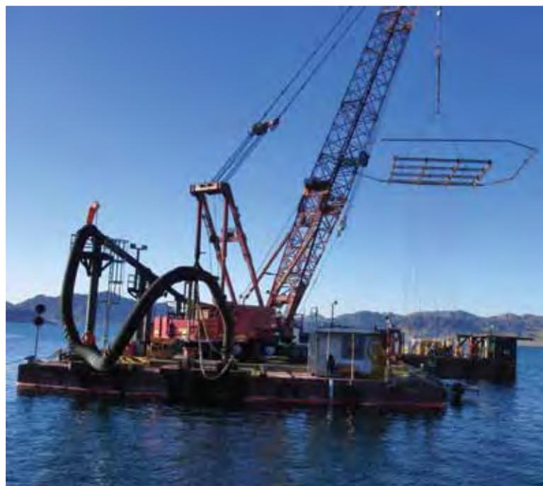
Lake Mead, the largest man-made reservoir in the United States, is located about 30 miles southeast of Las Vegas, Nevada. For the construction of Lake Mead's third water intake, which is entirely placed underground, an underwater excavation was needed at a depth of 100 m (330 ft): a large surface had to be deepened by 20 m (66 ft) in basalt.
