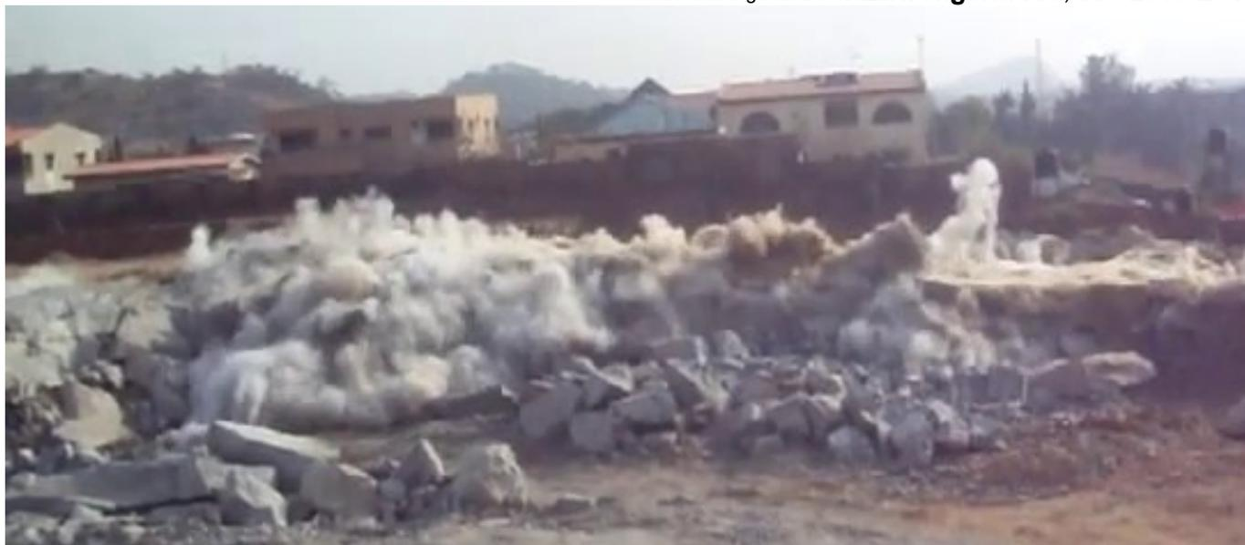
A 2500 m<sup>3</sup> in bench blast with of ground vibration and flyrock control
