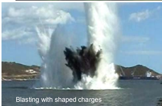
Blasting close to the old docks Control of the overpressure wave in water by means of air bubble curtaining
