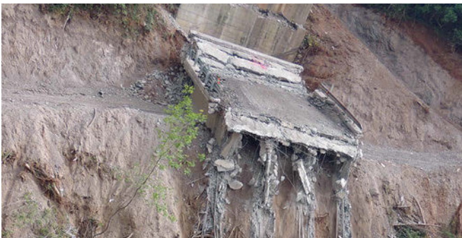
Figure 26. Spans more extensively demolished for better adjustment on the steel sloped footprint, to prevent its sliding toward the pylon below.
