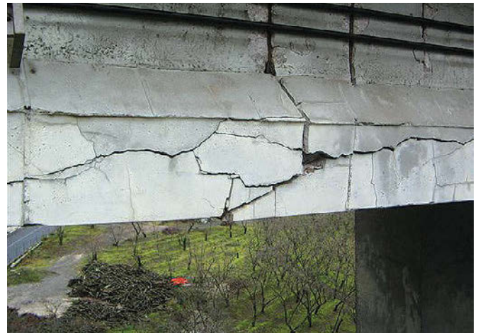
Figure 8. Large cracks in the lower bulb of a reinforced concrete pre-tensioned I girder.
