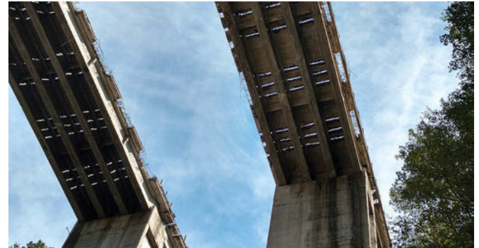
Figure 17. Spans ready to be blasted for extended explosives demolition due to constraints at footprint (steep slopes and structures to be safeguarded). I girder type (as bridges in figures 3-6).
