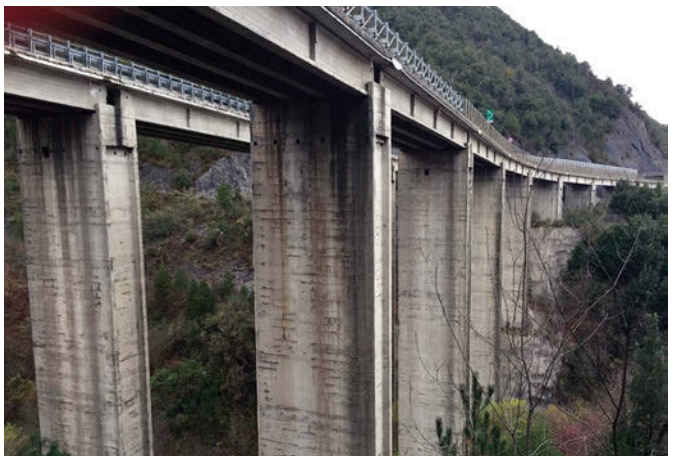
Figure 5. Bridge "Battendiero 1," Italy, 1970. Single box pylons for single 32 m simply supported spans four I girders carriageway.
