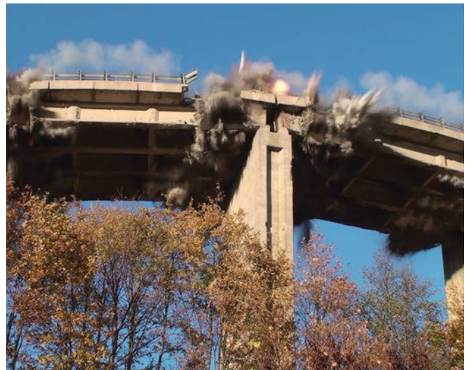
Figure 22. Spans and pylons blasted in sequence, safeguarding own pylons.
