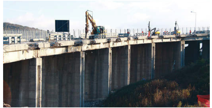
Figure 16. Preparing the spans to be blasted, by breaker on remote controlled excavator for preliminary decks demolitions and by remote controlled wagon drill for boreholes in the girders
