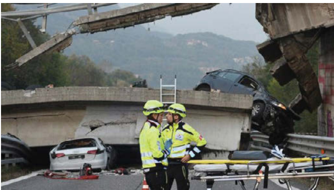
Figure 12. Collapse of a highway overpass causing casualties, 2016.
