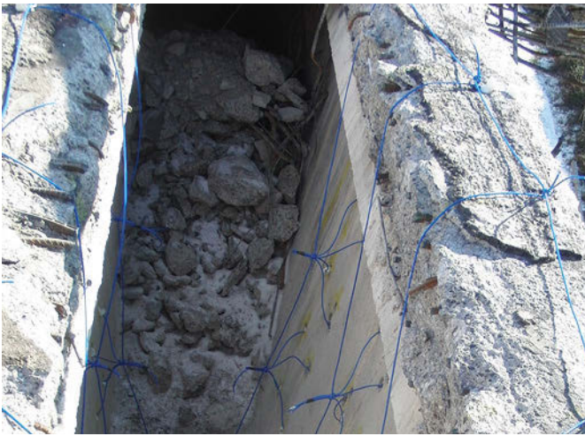
Figure 18. Spans ready to be blasted - box girder type (as bridge in figure 7).
