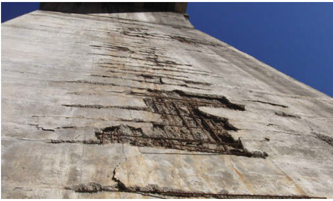
Figure 10. Reinforcement bars exposed and corroded in a box type concrete pylon.
