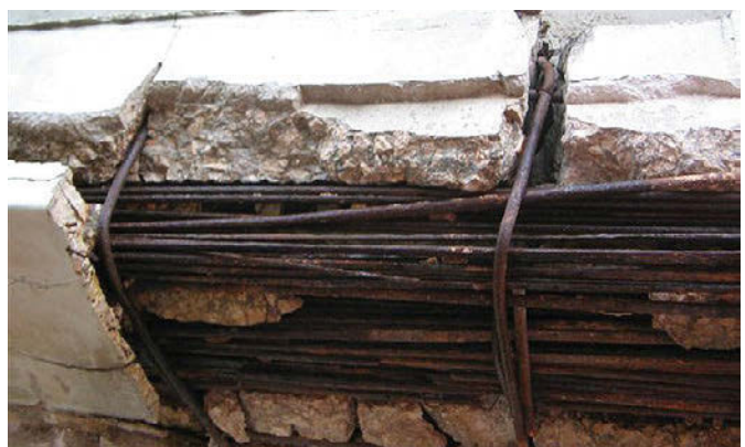
Figure 9. Re-bars and tensioning bars exposed and corroded after concrete cover collapse in the lower bulb of an I girder. Due to excessive re-bars, concentration concrete could not properly wrap around.
