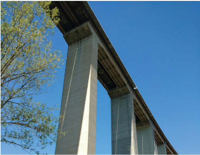
Figure 19. Spans to be demolished by safeguarding own pylons or with the new superstructure already in place built right above (before the blast).
