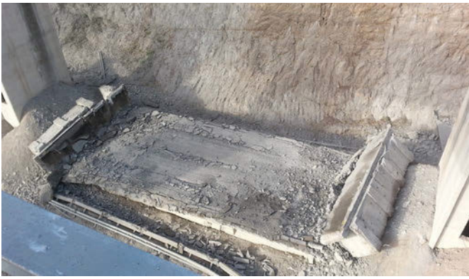
Figure 24. Heads of the girders from both sides of the spans are seen rotated and laying above the deck.
