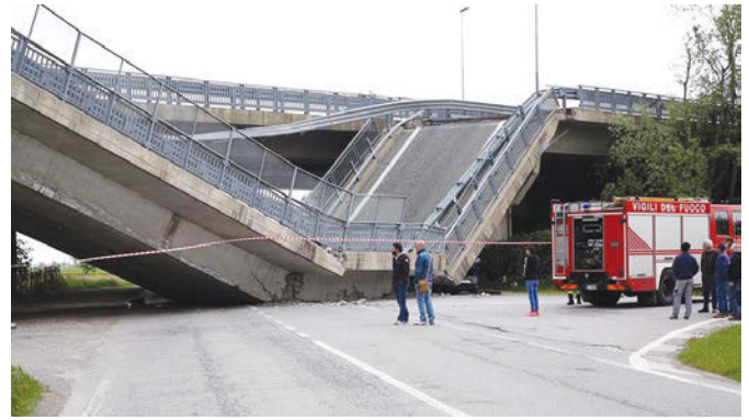
Figure 13. Collapse of a highway overpass causing no casualties, 2017.
