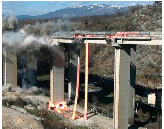
Figure 21. Spans and pylons blasted in sequence (redundant detonating cord circuit and firing sequence by redundant non electric detonators).
