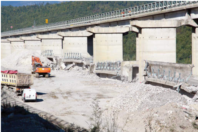
Figure 25. Span at the ground among own pylons. Collapse determined by hinging the beams close to their bearing spots.
