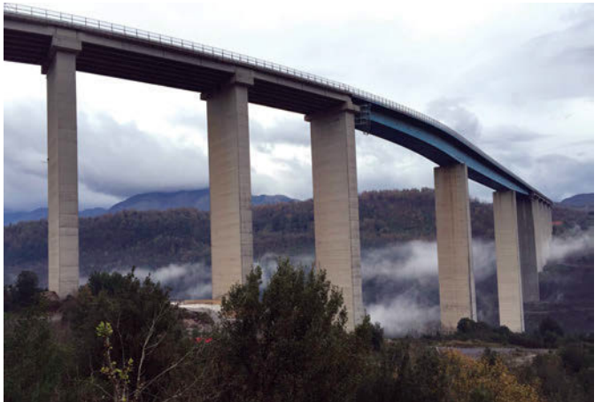
Figure 4. Bridge "Italia," Italy, 1968. Single box pylons with internal wall, carrying double 45 m simply supported spans four I girders carriageway.
