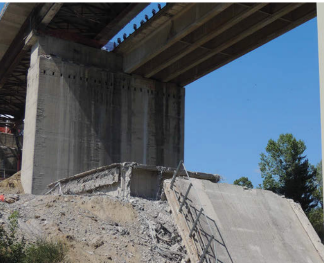
Figure 20. After the blast.
