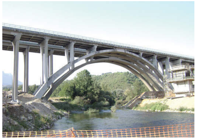
Figure 3. Bridge "Tanagro," Italy, built 1970. Reinforced concrete arch surmounted by twin full concrete pylons carrying single 32 m simply supported spans four I girders carriageway.
