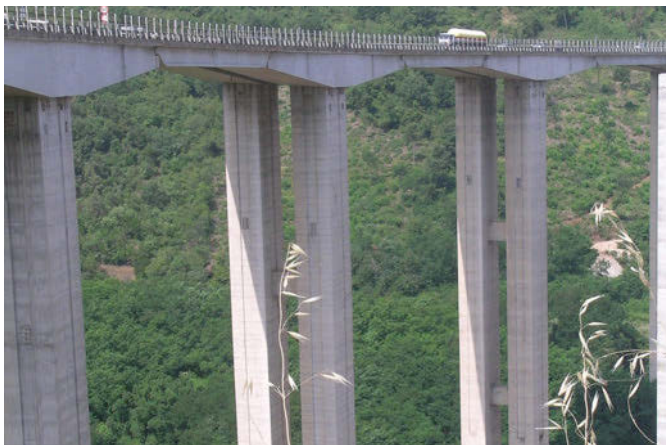
Figure 6. Bridge "Lontrano," Italy, 1968. Single thick walls box pylons with quadruple 25 m long cantilevers carrying double 32 m spans carriageways.
