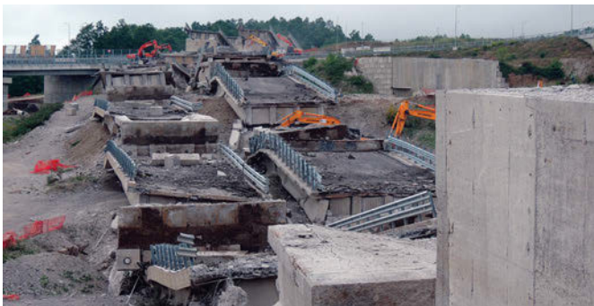
Figure 27. Spans and pylons at the ground, ready for mechanical breaking.
