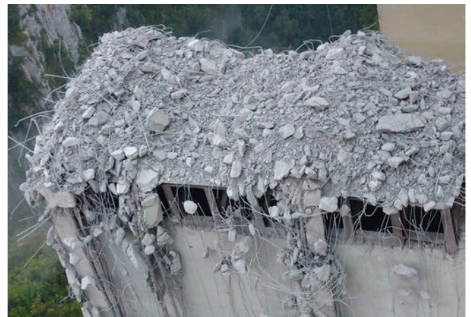
Figure 23. Concrete debris, re-bars and tensioning steel left from the extended explosives demolition of a 650 ton span overlaying this new pylon standing 17 meters right below it (see figure 17).
