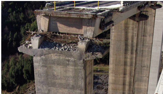
Figure 7. Bridge "Noce" Italy, 1970. Single thick walls box pylons carrying single 32 m spans carriageway double box girder.
